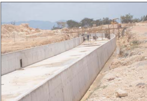
A drain under construction in Flankers near the Industrial Estate. The drain is being built as part of Segment 2a, of the North Coast Highway Project.
