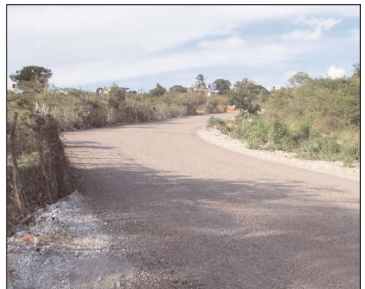
Completed section of the Red Dirt to Garlands main road, in St. James.
