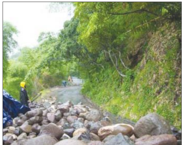
Stockpile of boulders to be used in constructing the retaining walls in Clarendon.
