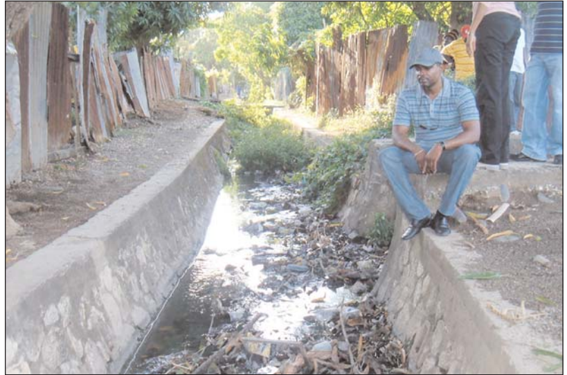
Major Projects Manager, George Knight looking at one of the drains in St. Thomas slated to be cleaned as part of the Disaster Mitigation component of the Special Flood Damage Programme.
