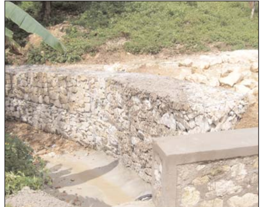
Completed Gabion retaining and head wall in Blackgate in Hanover.
