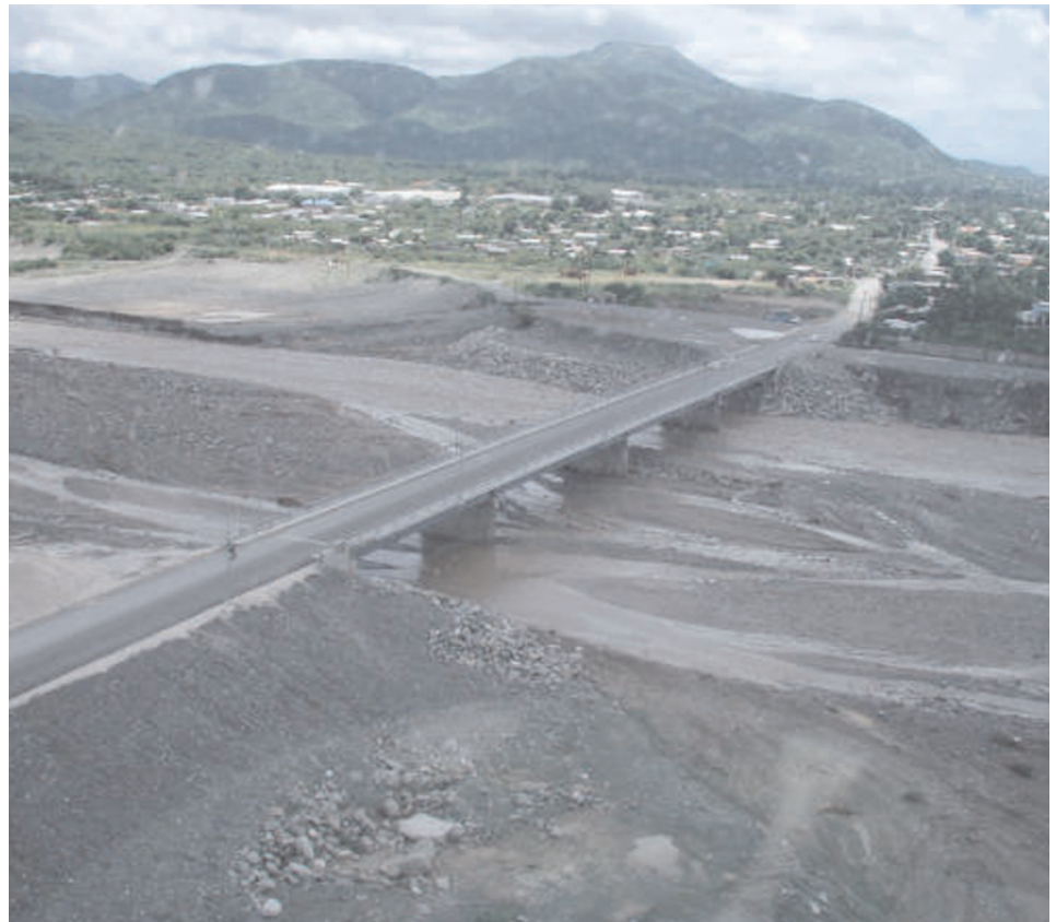
An aerial view of the newly constructed Yallahs Bridge, St. Thomas.
