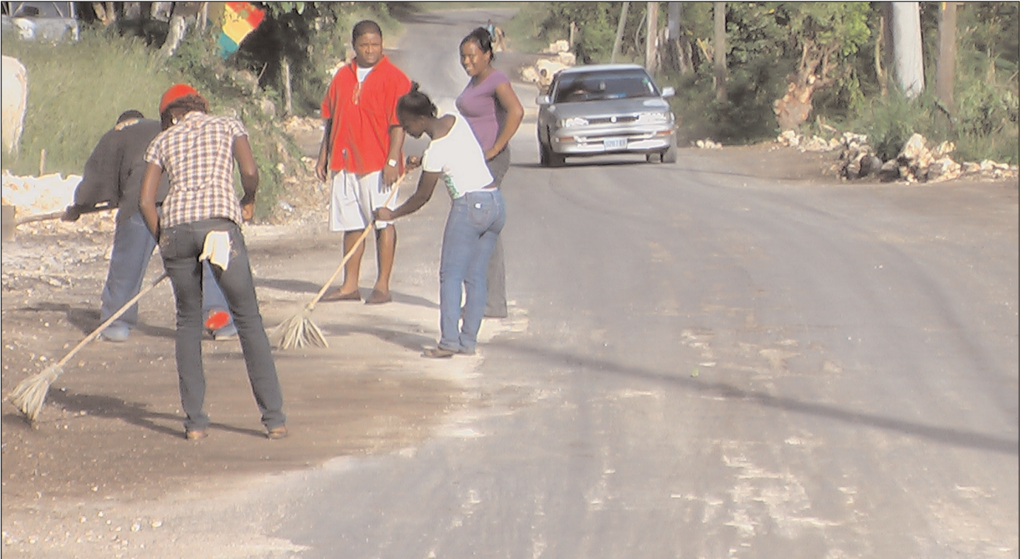
Workers sweeping loose material from a section of the Adelphi to Kent roadway in preparation for paving
