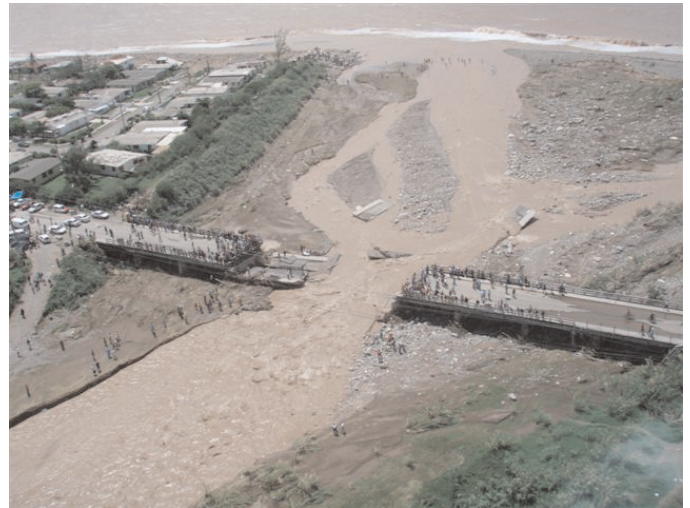
Aerial view of the Harbour View Bridge, St. Andrew after the passage of Tropical Storm Gustav
