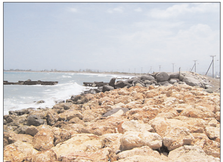
Photos show Rock revetment work done before the passage of Tropical Storm Gustav along the Palisadoes Road in Kingston.
