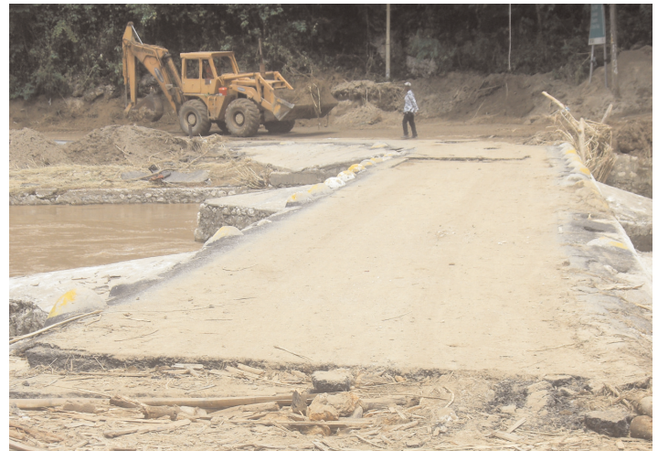
The Flat Bridge, St. Catherine after the passage of Tropical Storm Gustav
