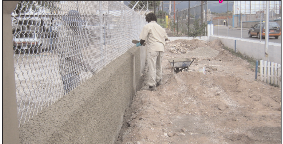
Workmen applying the final touches to a boundary wall along Dunrobin Avenue
