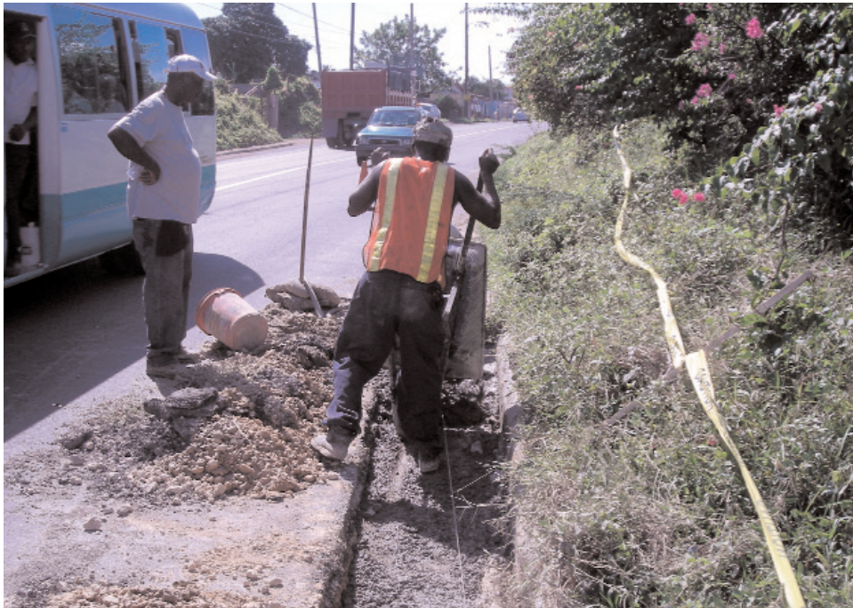
Workmen construction a side drain along the Gutters to Freetown Main Road
