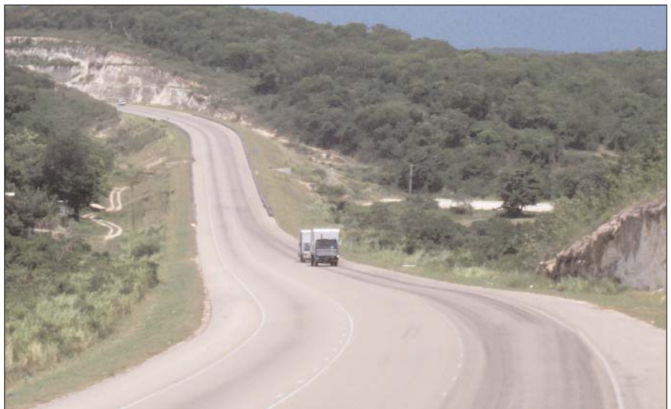
A Section of Segment II of the Northern Coastal Highway
