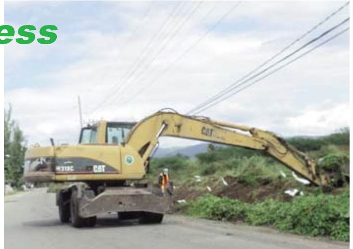
Drain cleaning along the Jacob Hut to Milk River Road
