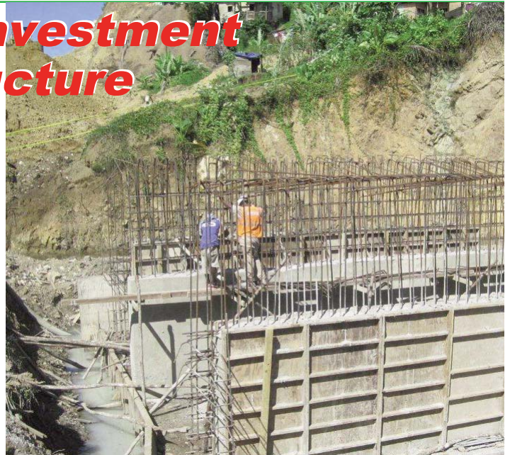
One of the two Box Culverts under construction at Johns Hall, St. James
