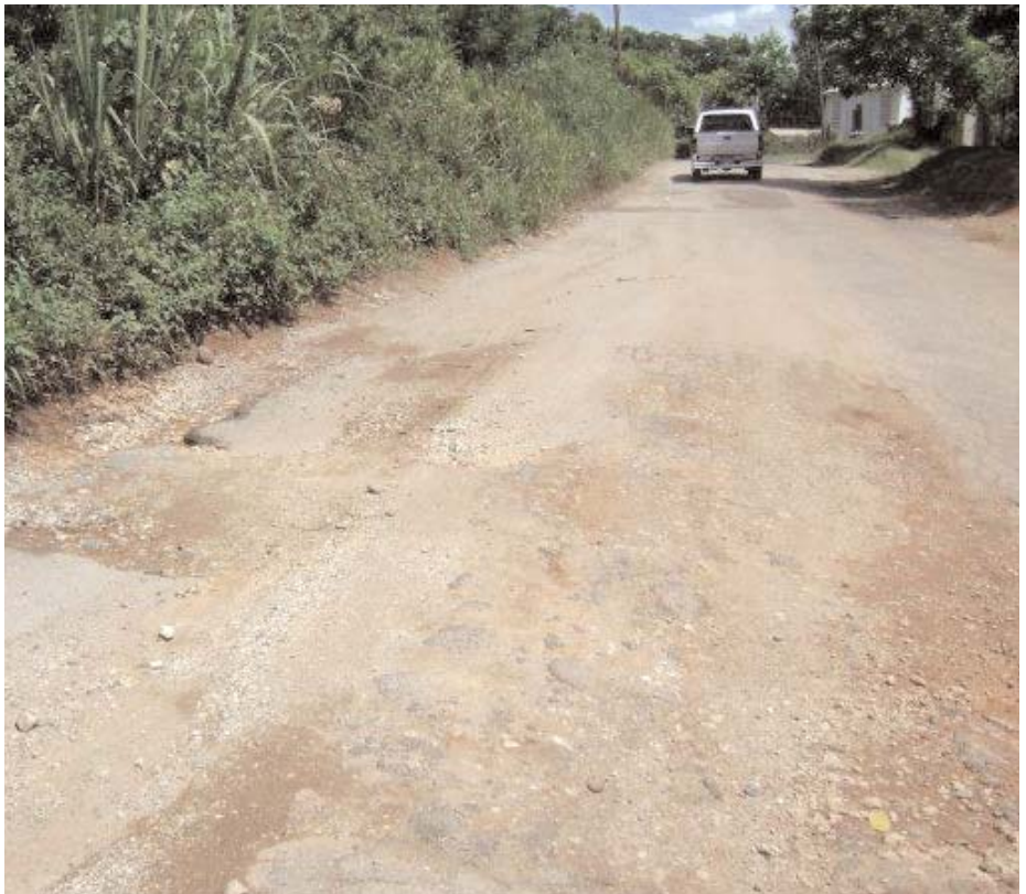
Badly rutted section of the corridor
