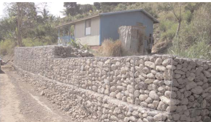
Gabion Wall along the Lower Chapleton main road
