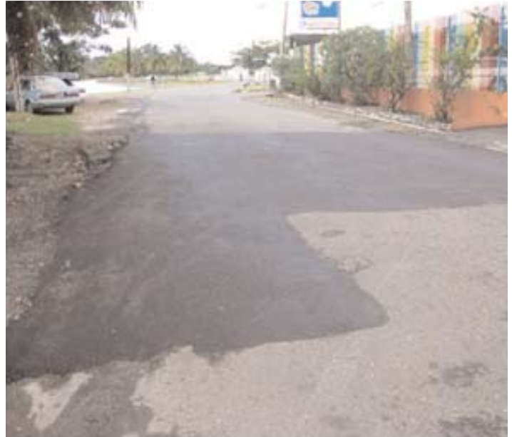
A completed section of the Folly – Hector's River main road
