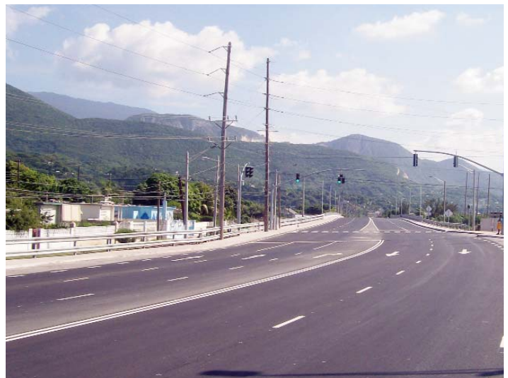
A section of the New Dry River Bridge and Harbour View Main Road
