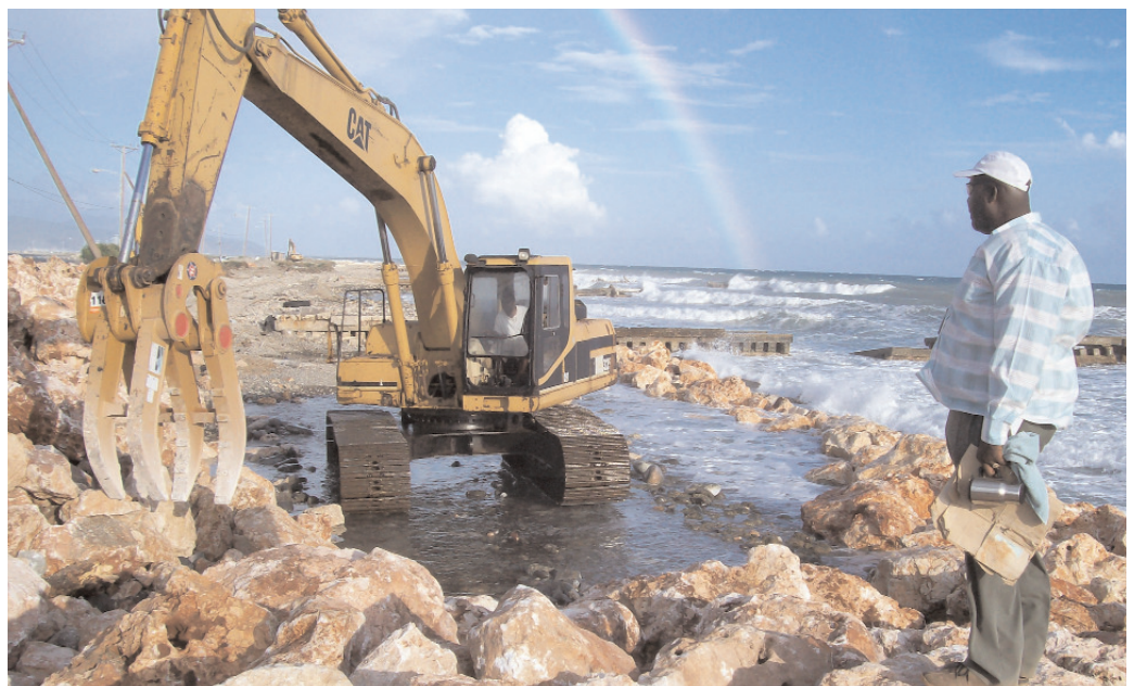
"Put that one right there!" Clerk of Works, Caswell Whyte monitoring the placement of rocks along the Palisadoes Road. The rock revetment (wall) is being constructed along the strip to assist in mitigating the effects of high tide and wind, which often results in sections of the road becoming impassable.
