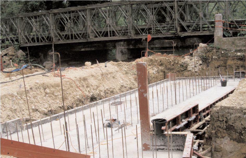
Foundation for one of the abutments of the new Steel Girder Bridge, Seven Rivers, St. James.
