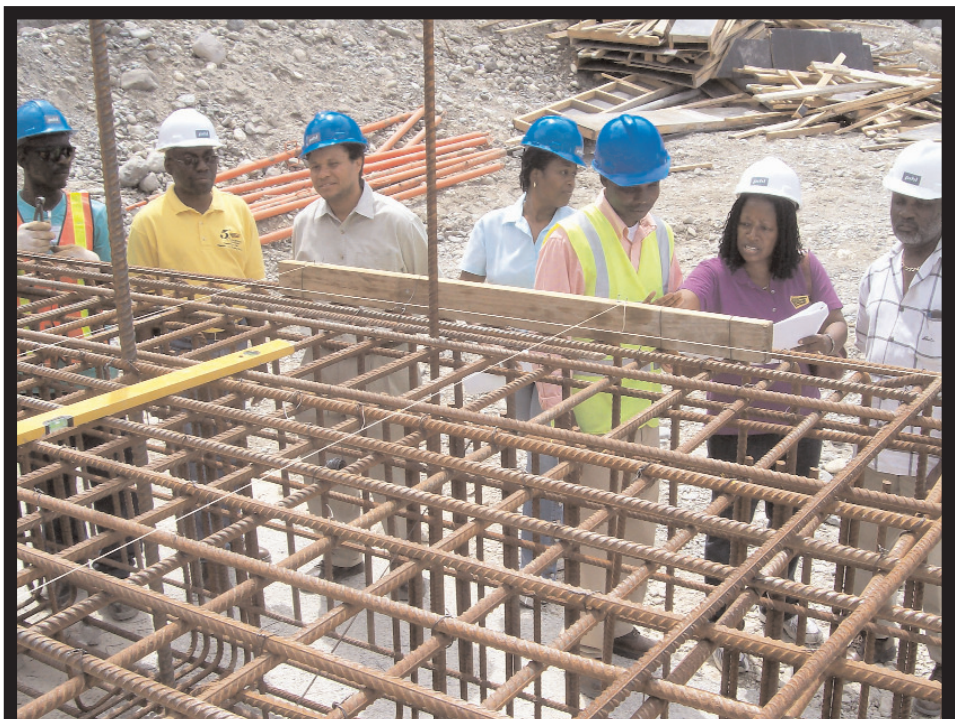
This is how it is done - by staff! Director of Human Resources Management and Administration, Jennifer Henry (second right) pointing to the plan for the western abutment at Yallahs, St. Thomas
