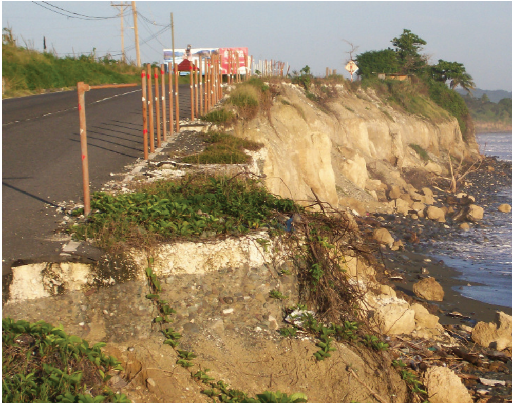
Roselle main road. This section of road is slated to undergo major rehabilitation as part of the US$10 - million programme
