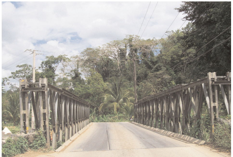
The existing Bailey Bridge which will be replaced.
