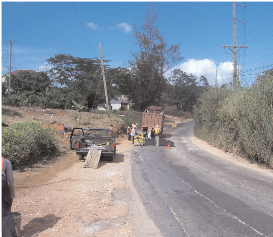
Patching exercise underway along the Spur Tree main road in Manchester.
