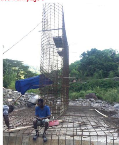
A resident of Chesterfield, St. Mary employed to the bridge works, sits atop steelwork observing another worker tying steels in preparation to bring the bridge's centre pier above its foundation.
