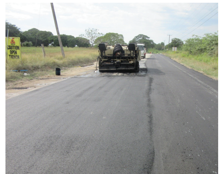
Application of wearing surface
