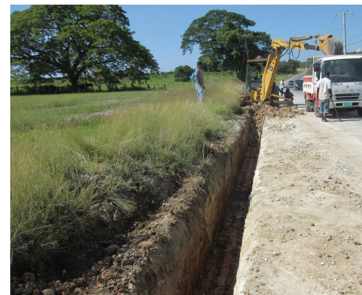
Excavation to facilitate the laying of pipelines
