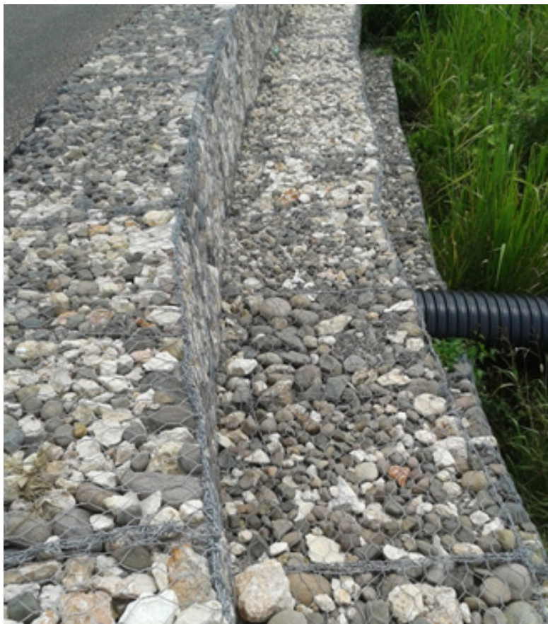
A section of the Wait-A-Bit to Joe Hut roadway where a Gabion retaining wall was constructed.
