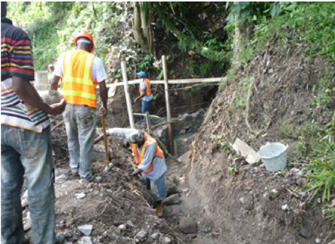
U-drain under construction
