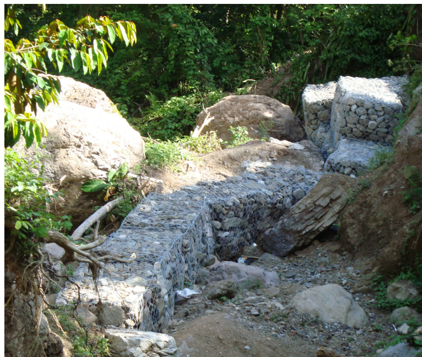
The placement of Gabion baskets commencing reconstruction of the road in Nedhut, St. Andrew
