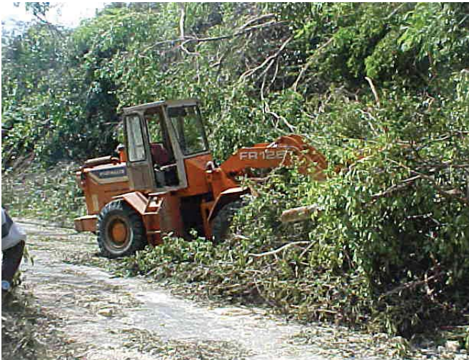
Loader cleans fallen trees along the Hopton to Auchindown main road, Westmoreland.
