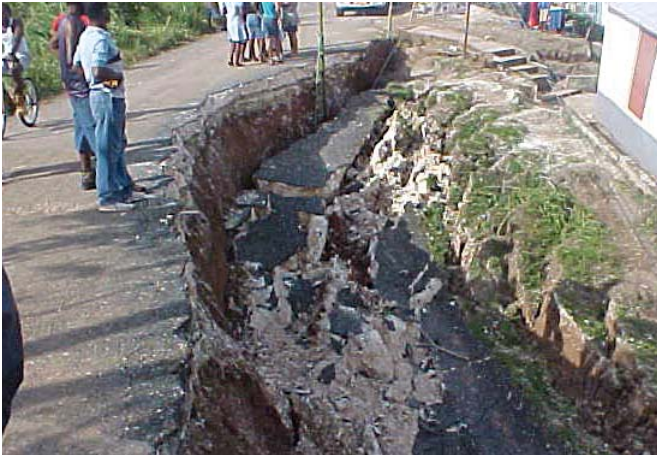
Damaged section of the Point to Flamstead Gardens main road at Tangle River, St. James.
