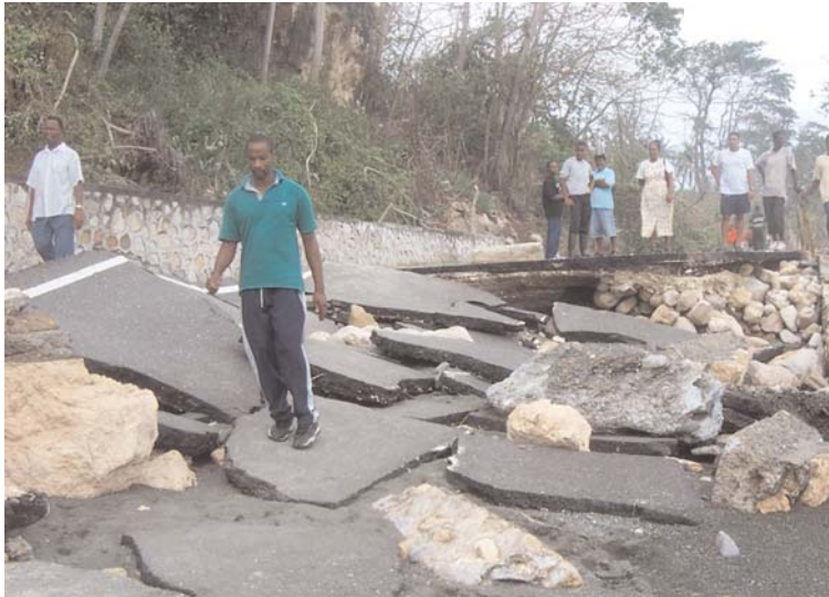
Roselle main road, St. Thomas, extensively damaged during the passage of Hurricane Ivan.
