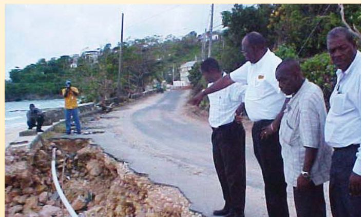
State Minister for Transport and Works, Hon. Dr. Fenton Ferguson (2nd left) points to a breach in the sea defence structure along the Manchioneal main road in Eastern Portland. Looking on are L-R Member of Parliament Dr. Donald Rhodd, resident and Mr. Winston Palmer, Parish Manager - Portland
