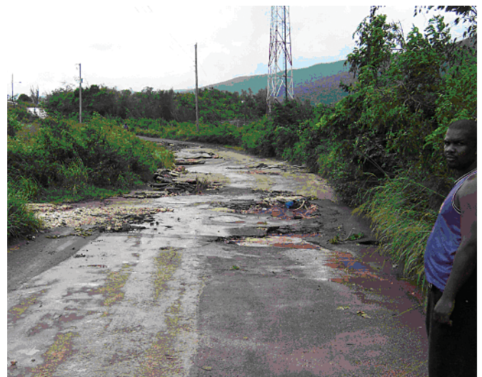
This section of the Downs to Alligator Pond main road in St. Elizabeth was badly scoured during the passage of Hurricane Ivan.
