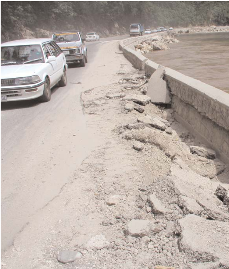
A section of the road, which leads to the Flat Bridge that was damaged during Hurricane Ivan.
