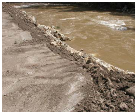
Damage section of Bog Walk Gorge in St. Catherine.
