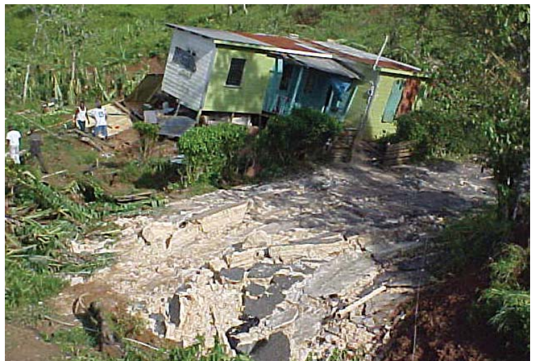
Another damaged section of the main road leading from point to Flamstead Gardens in St. James.
