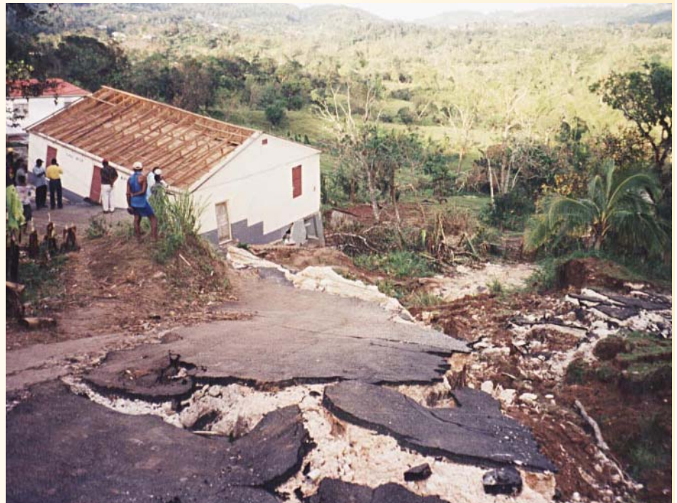
Damaged roadway, Tangle Rive, St. James
