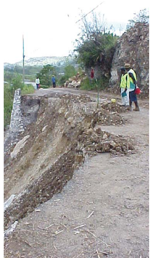
This section of the Sandy River to McNie via Rhoden Hall main road in Clarendon was badly damaged during the passage of Hurricane Ivan.
