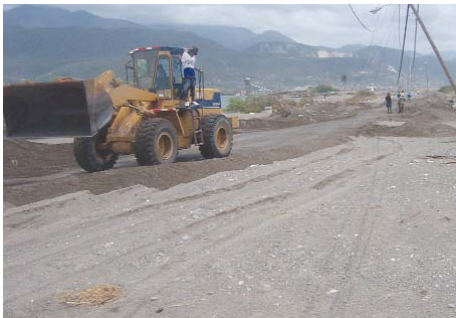
Palisadoes - Front-End Loader removing sand that covered the Palisadoes main road.
