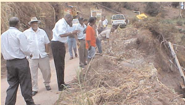
State Minister for Transport and Works, Hon. Dr. Fenton Ferguson (3rd left) makes a point as he inspects a huge breakaway at Section in Portland.
