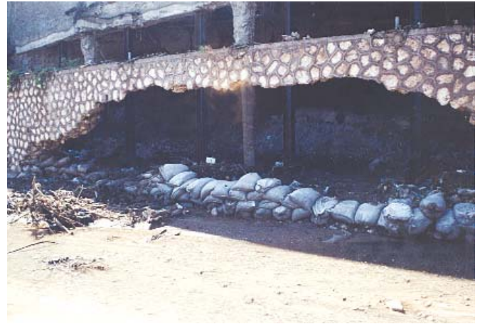
A section of the Sandy Gully retaining wall, adjacent to the Trade Centre, damaged during Hurricane Ivan.
